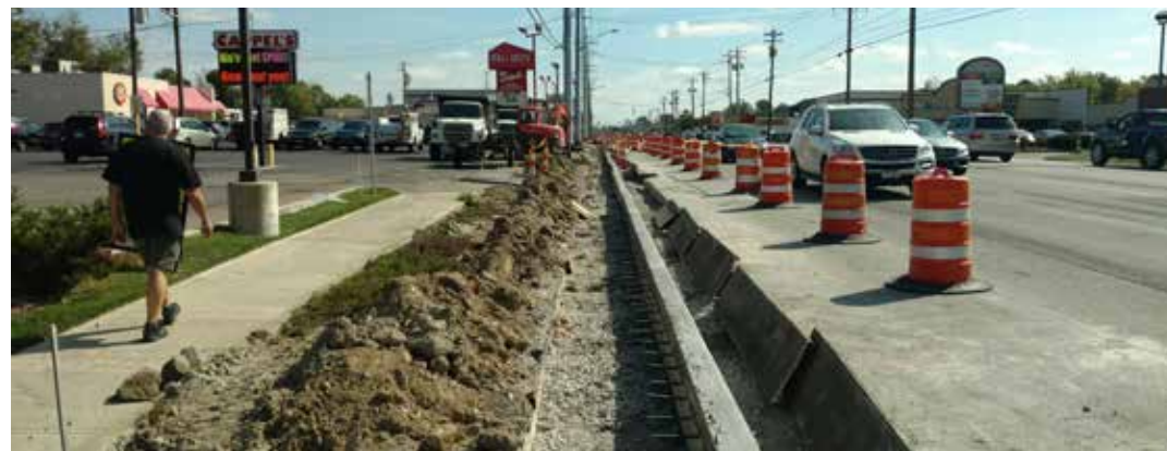
Construction in the Downtown Anderson area
